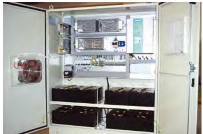
Emergency power system BBU
